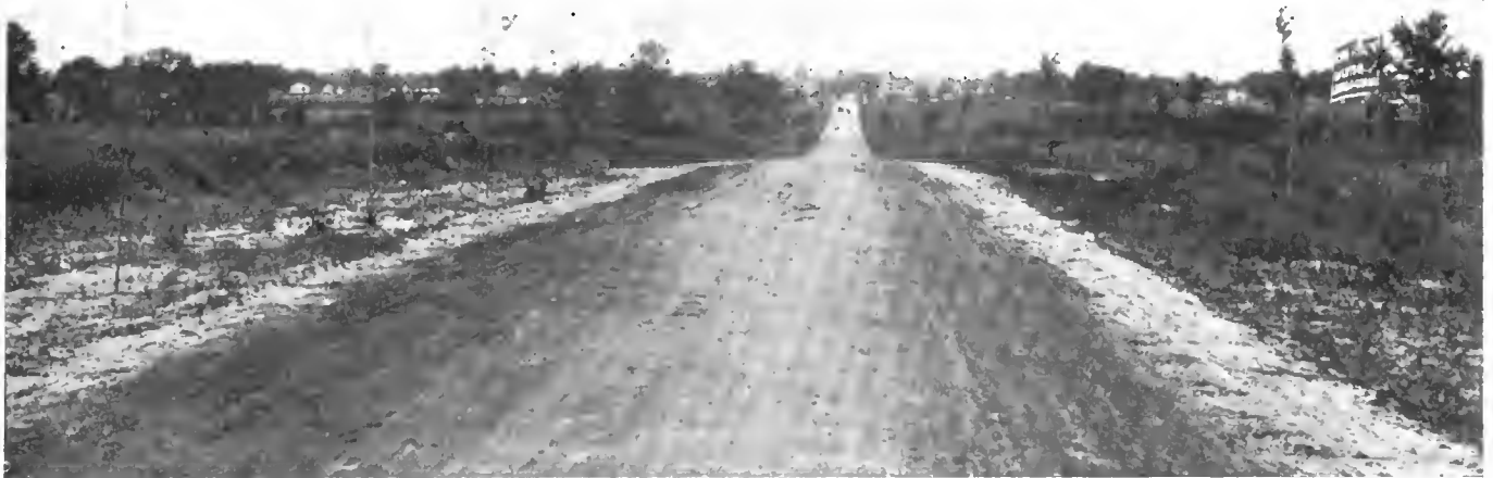
Experimental Stretch of Coal Tar Treated Road at Savannah, Ga., on Henry Street, Looking Westward into the Suburbs.
